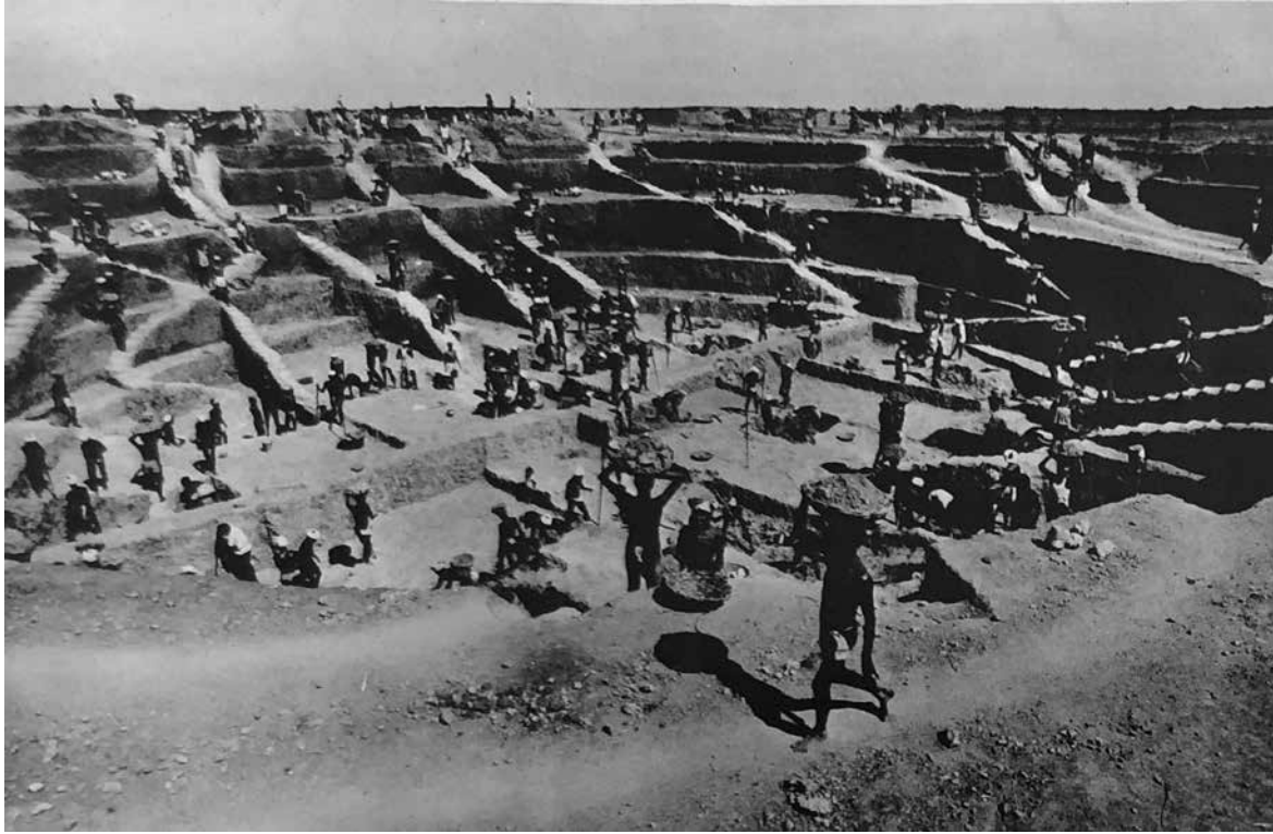
Construction work at Matrimandir
