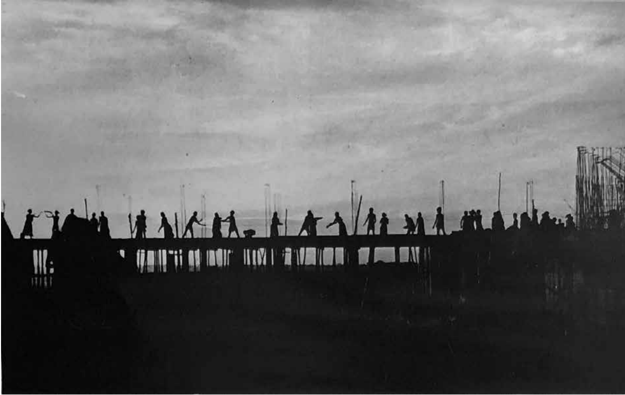
Auro-Dairy under Construction
